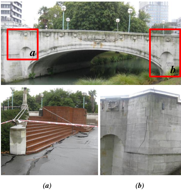
Figure 6: Bridge of Remembrance (a) Damage to steps on western approach [Courtesy of Opus]; (b) Damage to north-eastern wingwall [Courtesy of Opus].
