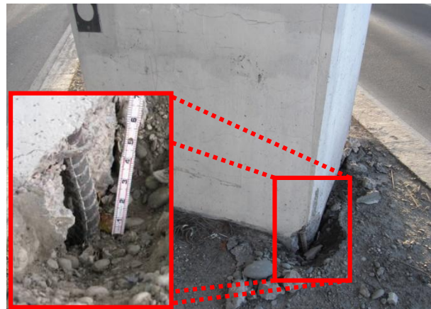
Figure 21: Port Hills Overbridge. Buckling of reinforcing steel at the base of the piers [Courtesy of Opus].
