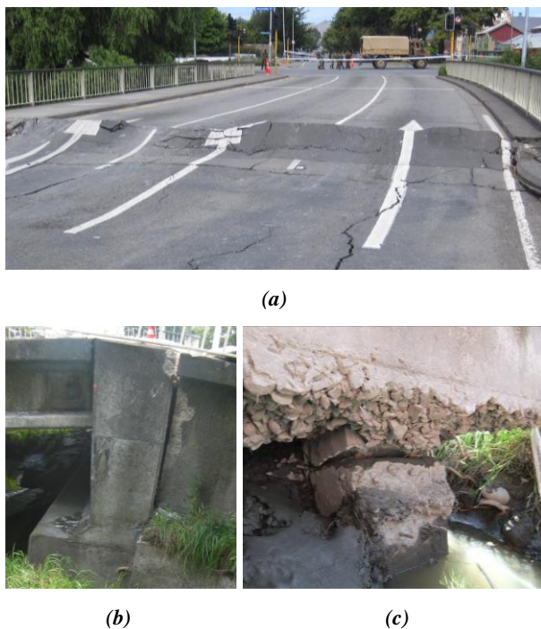
Figure 16: Fitzgerald Avenue Bridge (a) Damage at the approach of the eastern bridge [Photo by A. Kivell]; (b) Back-rotated abutments [Courtesy of Opus]; (c) Flexural cracks on the piles [Photo by L. Hogan].
