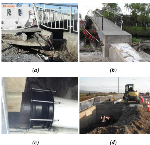
Figure 22: (a) Gayhurst Road Bridge, damage to lifelines [Photo by A. Palermo]; (b) Dallington Pedestrian Footbridge, damage to electrical services to the Dallington area [Photo by M. Le Heux]; (c) Repair to water pipe at Bridge Street Bridge [Photos by A. Campbell]; (d) Repairing works at Bridge Street Bridge [Photo by A. Palermo].
