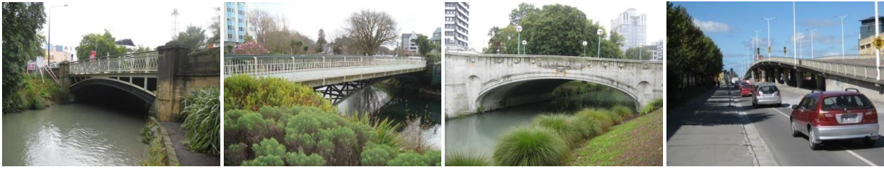
Figure 4: Selection of damaged bridges in the CBD area. From left to right: Colombo Street Bridge; Bridge of Remembrance; Antigua Street Footbridge; Moorhouse Avenue Overpass.
