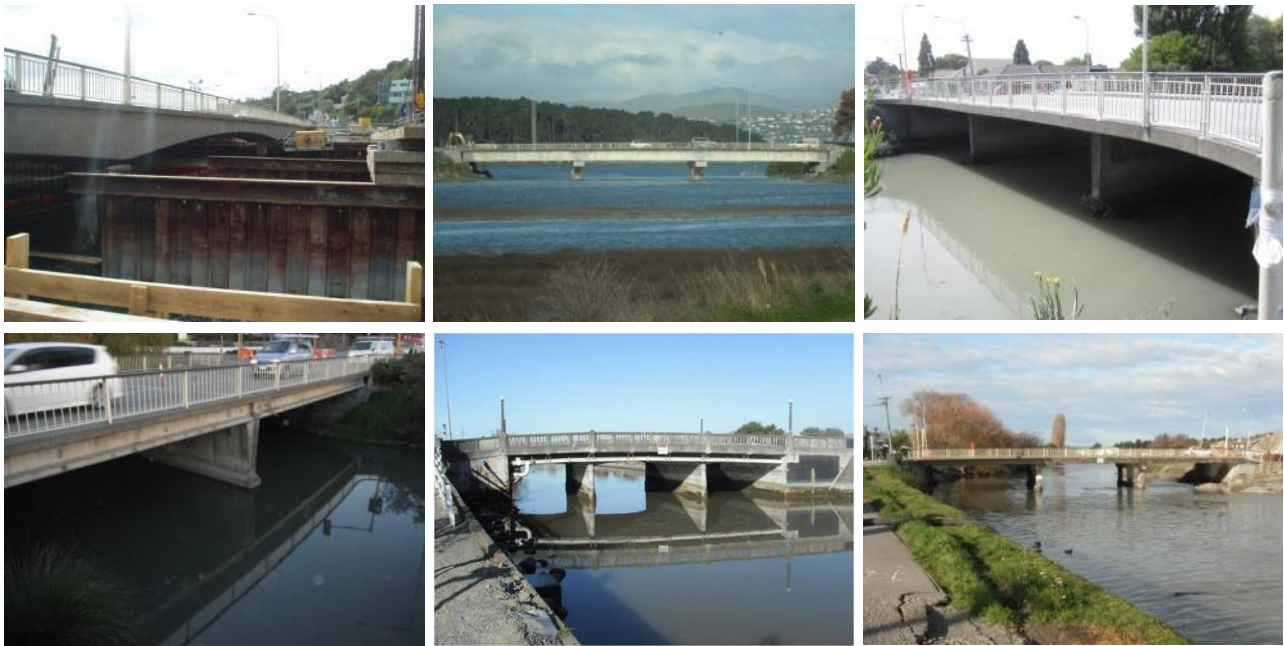
Figure 12: Selection of damaged road bridges. Clockwise from top left: Ferrymead Bridge; Bridge Street Bridge; Gayhurst Road Bridge; Avondale Road Bridge; Pages Road Bridge; Fitzgerald Avenue Bridge.
