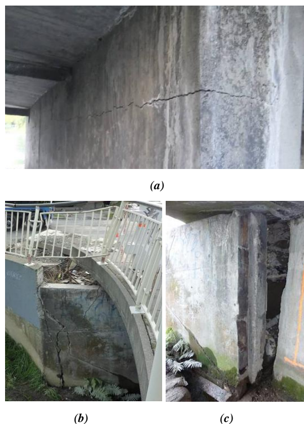
Figure 15: Gayhurst Road Bridge (a) Damaged pier with flexural cracking [Photo by L. Hogan]; (b) Flexural cracks at the north-western wingwall [Photo by L. Wotherspoon]; (c) Displacement of north-western wingwall [Photo by L. Wotherspoon].
