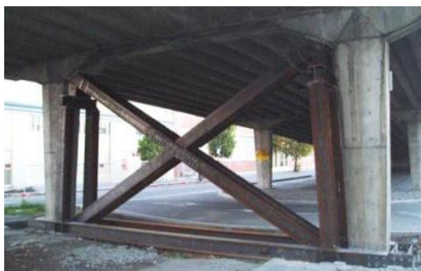
Figure 11: Moorhouse Avenue Overpass. Temporary propping [Photo by G. Whiula].
